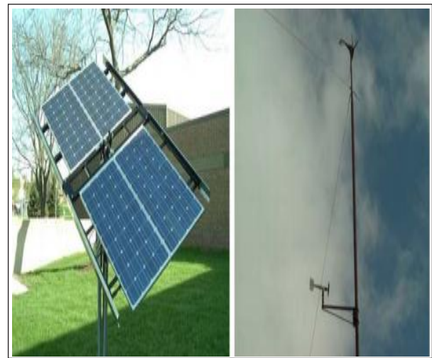
Fig. 1: Existing 1.5 kW Wind Solar Hybrid Power Unit Interface of the Wind Solar Power System
